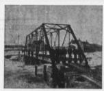
STEEL HIGHWAY BRIDGES. CONCRETE ABUT-MENTS. REINFORCED CON-**GRETE FLOORS**
