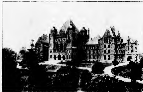
ONTARIO PROVINCIAL BUILDINGS, TORONTO.
