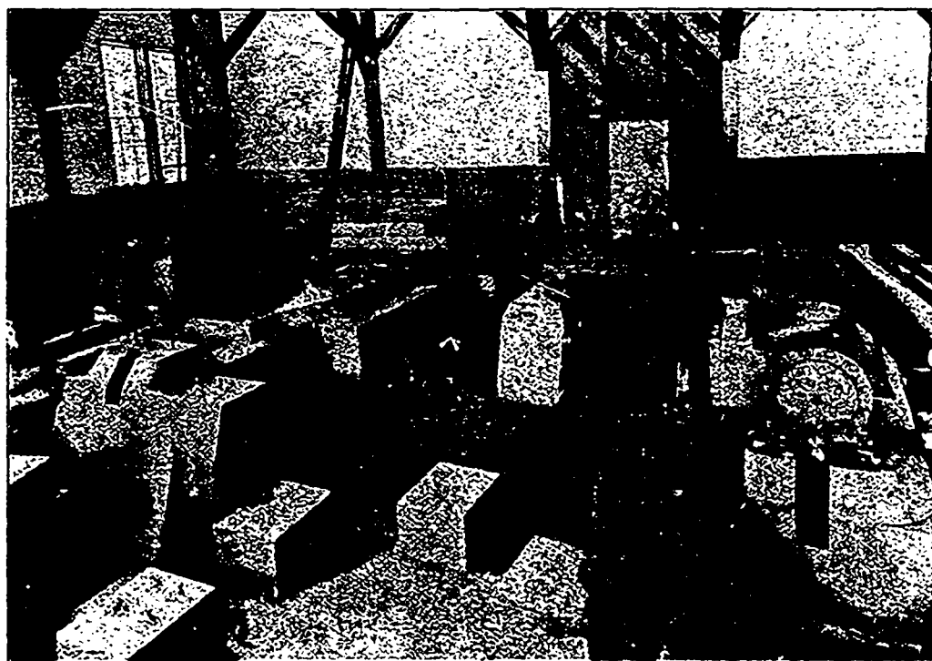
Concrete Foundation ready to receive General Traffic Hoist.
