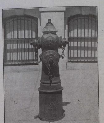
Fig. 1.—Type of Three-way Hydrant used in New Distribution System.
