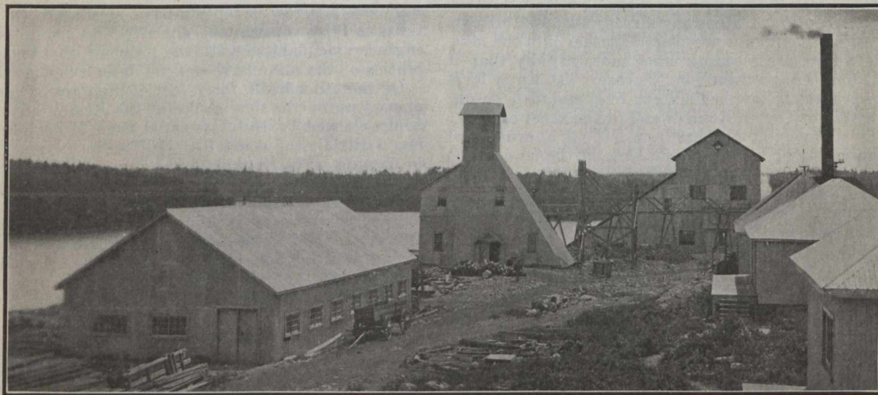
General View of Plant, Swastika Mine, Ont.
