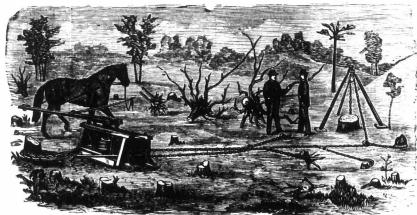
Two men and one horse only are required to operate this machine. Will pull green grubs and stumps ranging from three to twenty-four inches in diameter, and in many cases much larger, and any size with a little help. County rights for sale. The derrick as shown in cut is used only when very large stumps are to J. BARTON, P.O. Box 345, Toronto, Can.
