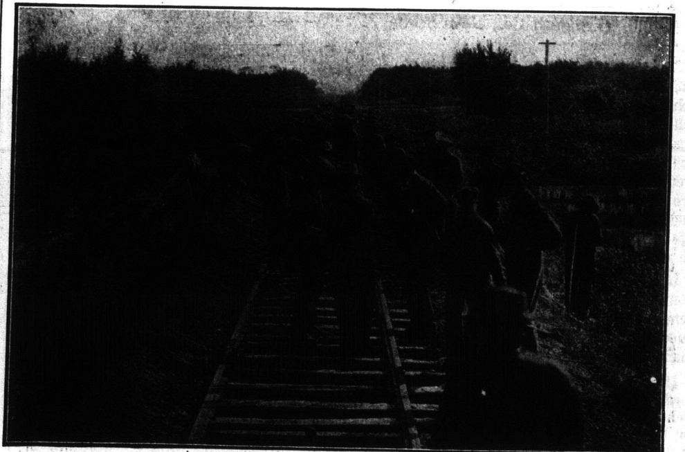
Ballasting track. C.N.R. construction.
