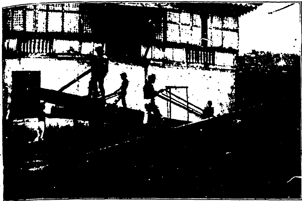
FIG. 3.—NATIVE METHOD OF SAWING TIMBER. THE NATIVES FIND THIS PRIMITIVE METHOD OF SAWING PROFITABLE EVEN WHEN COMPETING WITH A STEAM SAW MILL.
