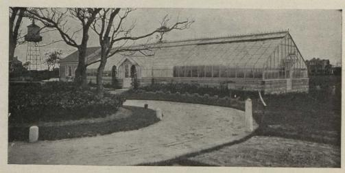
Last month our chat was particularly about the way these houses are bound to outlast others, because of no joints at the eaves, and the complete protection from decay of the wood in the steel encased U-Bar, but we stopped talking just as we were about to mention the question of heat.
