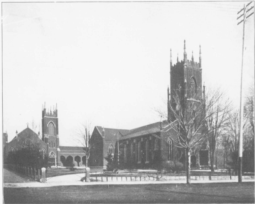
ST. PAUL'S CATHEDRAL AND CRONYN HALL (VIEW FROM RICHMOND STREET)
