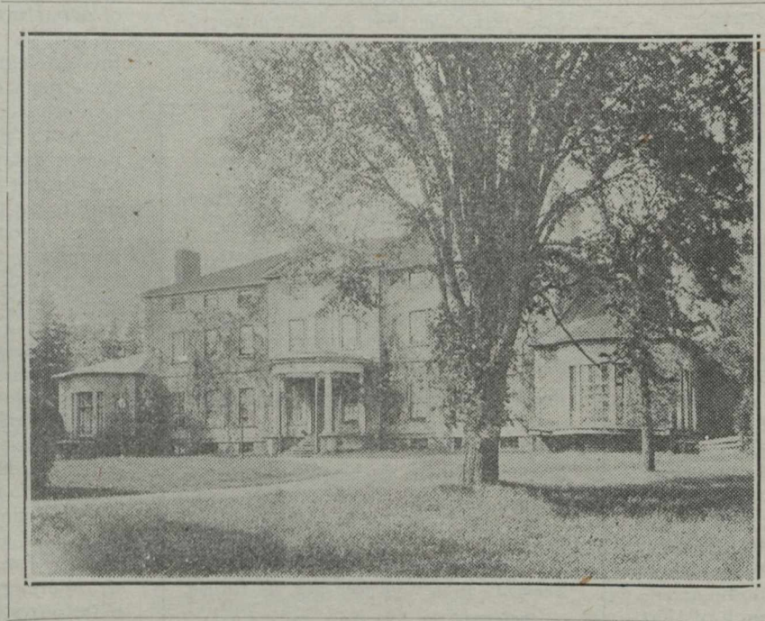
OLD GOVERNMENT HOUSE BARRACKS
