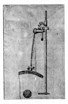
stroke or any length of diagram. The reduced motion relative to that of the piston is the same in every part of the stroke. The lever may be of any length between half stroke of the engine and four. times the stroke, with diagrams of any length Four indicadesired. tors can be operated simultaneously. Indicator strings leave the reducer at any angle. It is steady at all speeds of engine, and durable. One, with care, will last any engineer his life-time. Average weight, 4 pounds.
