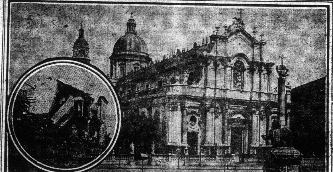
RUINS AT MESSINA, AFTER EARTHQUAKE. FAMOUS OLD CATHEDRAL AT CATANIA, THAT WAS DAMAGED.
