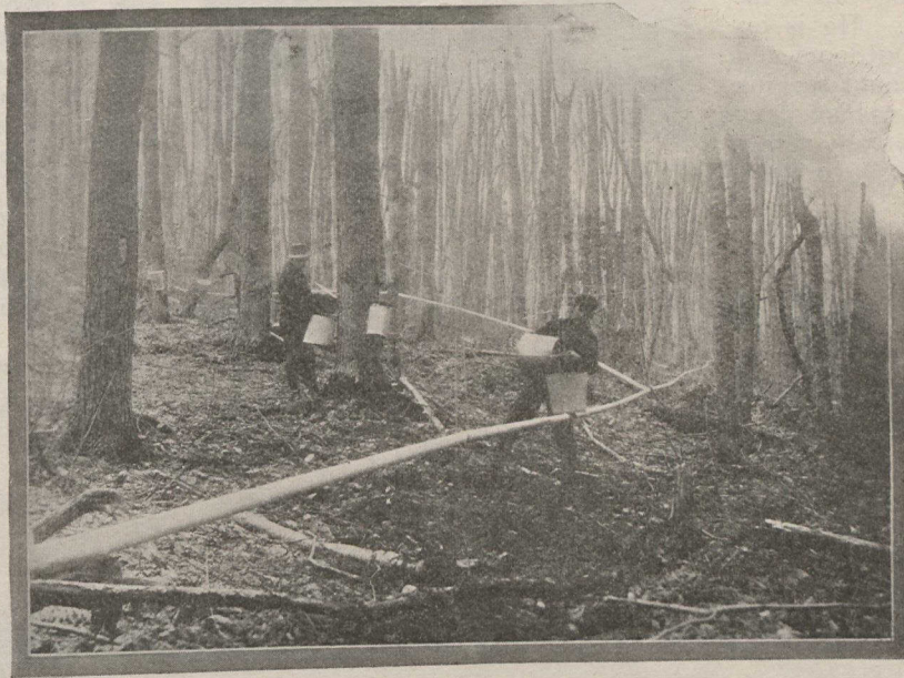
Through metal pipes the sap flows from the bush to the sugar house. Such equipment is being more and more adopted by the progressive maple bush owner where the size of his business warrants it.
