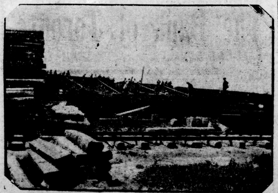
The sliding a short distance this side of St. Thomas, where thousands of tons of steel rails, required on the road, have been stored.
