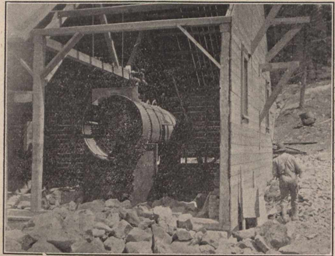
BOILER ON WHITE RESERVE MINE.
