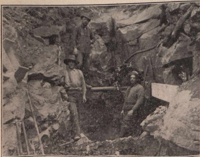
ROCK DRILL IN CUTTING, WHITE MINE.
