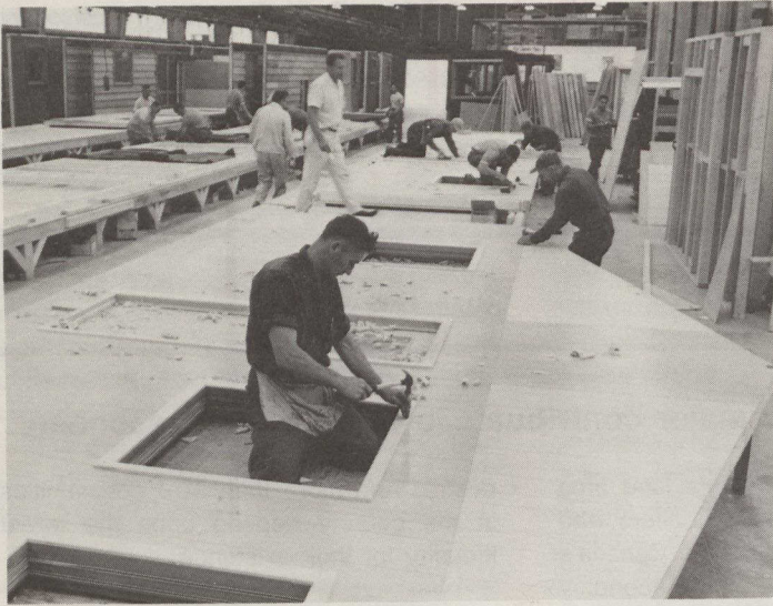
Construction workers prepare pre-fabricated houses for expanding national and international markets.
