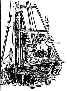
on land or water by Steam Pile Drivers or Drop Hammers.
