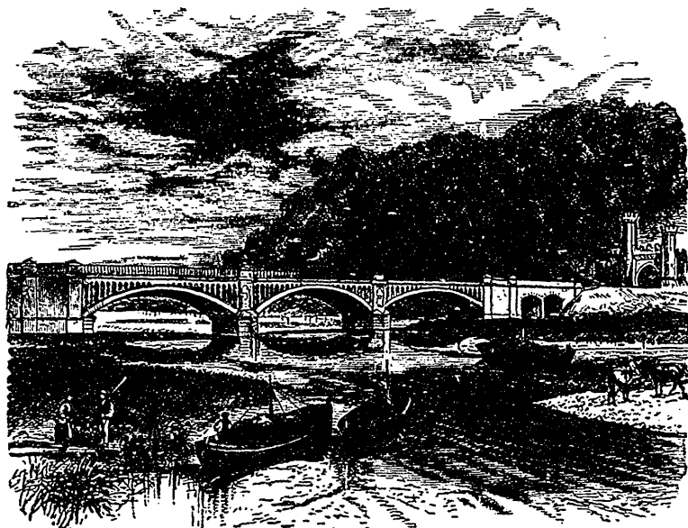
BRIDGE OVER THE TRENT.
