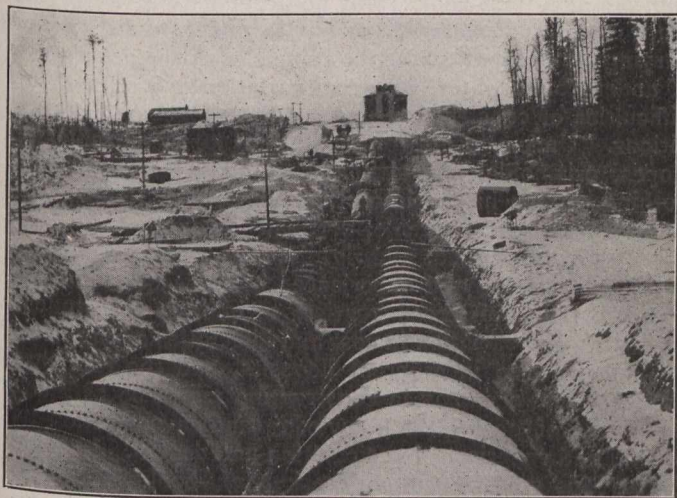
Two 8-ft. Iron Pipes, 1,300 ft. Long, from Surge Tank (in distance) to Power House at Wawaiten Falls.
