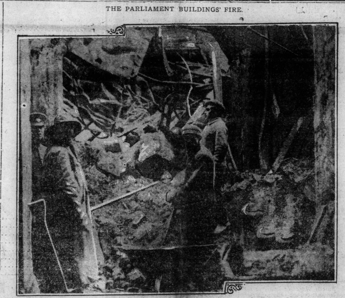
Digging for bodies in the main corridor at the point where the Clock Tower fell in. Here was found the body of Deputy Clerk LaPlante just before the Photograph was taken.
