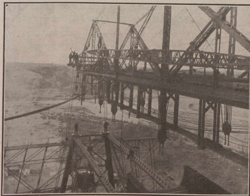
Fig. 21.—Cantilever Arm of Traveller. Note the erection cage suspended at the top of the tower.
