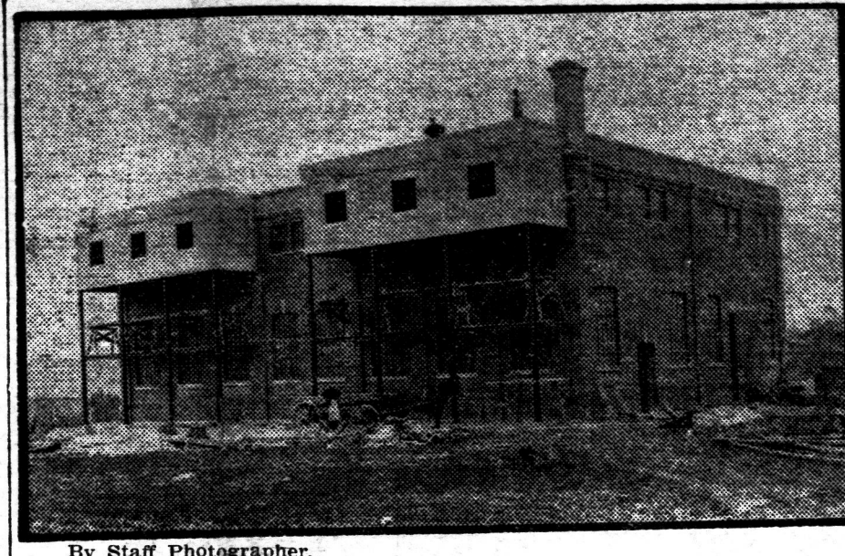
By Staff Photographer. THE HYDRO-ELECTRIC TRANSFORMER STATION. The building is situated south of the Hamilton road, and east of the city. Power will there be stepped down before it is sent into the city. By Staff Photographer.
