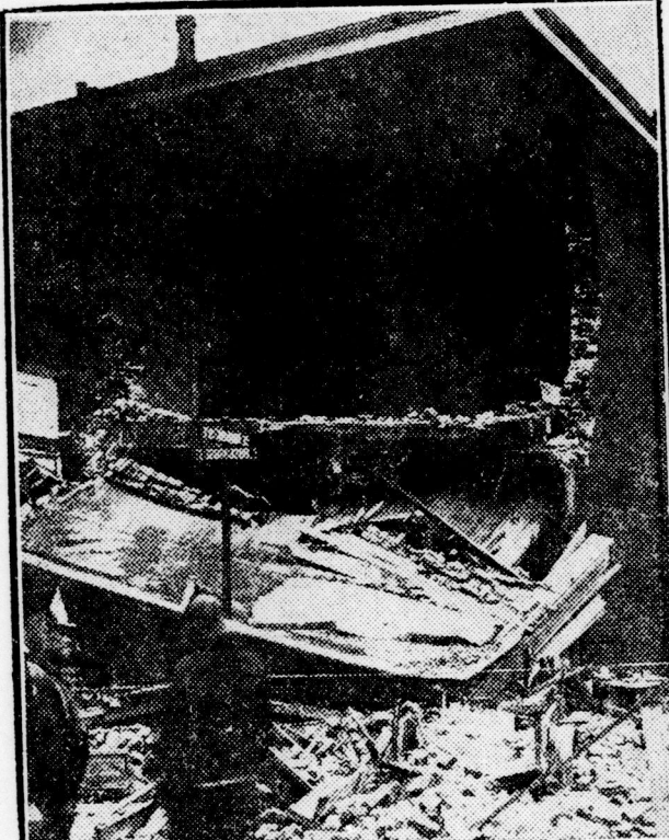
Sounds like a "whopper" to say that all this havoc was caused by a single motor truck, but it's a fact nevertheless. The heavy truck struck a supporting pillar of the building and the whole front of the structure collapsed
