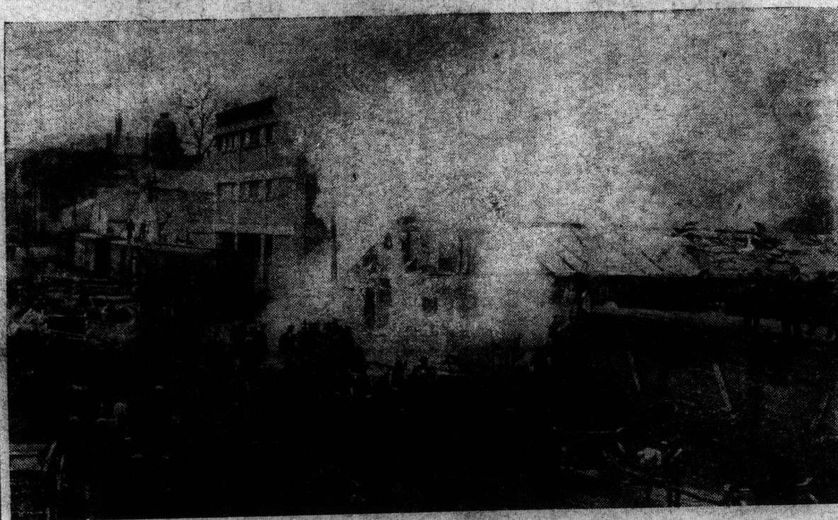
The above is the scene of last night's fire on Colborne street, when the Anguish livery barn was destroyed by fire. The building was one of the city's landmarks, and will be replaced by a modern structure.
