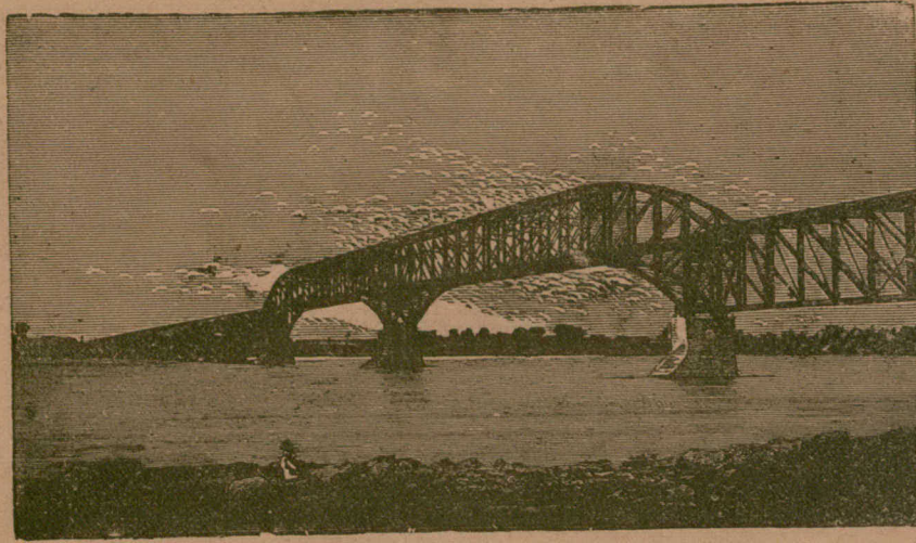
ST. LAWRENCE RIVER BRIDGE, CANADIAN PACIFIC RAILWAY, LACHINS, P. Q.
