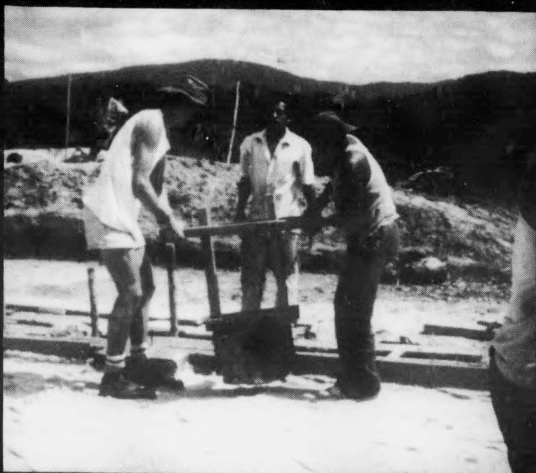
Preparing a foundation for a community health centre.
