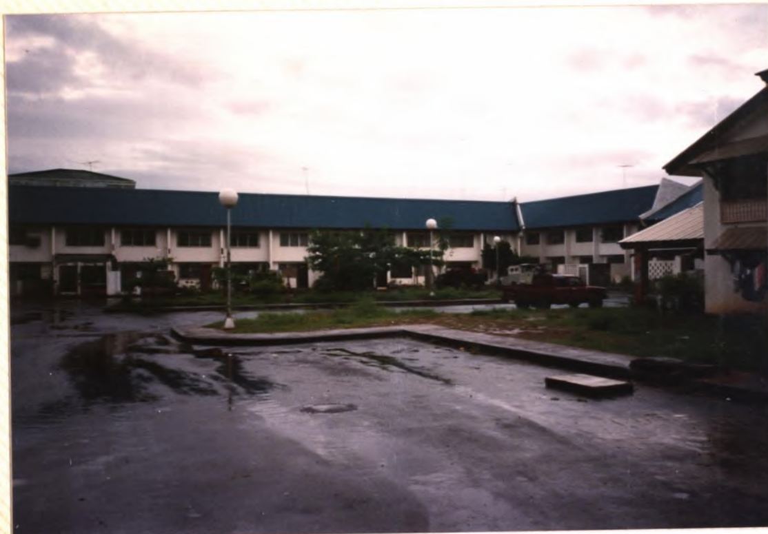
No. 54. Capitol BLISS townhouses. Each two-storey unit contains 79 sq.mtrs. floor space and sells for C$18,300.
