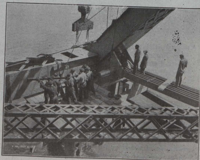
Fig. 4.—Driving Pin Connecting Bottom Chord Eye Bars at XLo Joint
