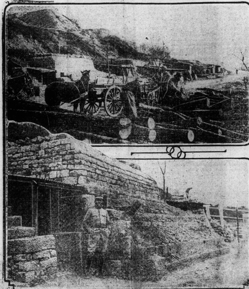
These pictures show the Cagnas (soldiers' houses) bombproof even under heavy shelling, and the bringing up of materials for new trenches. The strength of the French defences outwitted the foe.—(Exclusive Courier Pictorial Service, in conjunction with the London Daily Mirror.)
