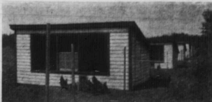
Row of Open-Front Poultry Houses at the Alberta Poultry Station, Edmonton. In winter the openings are closed with cotton. No glass is used in the construction.
