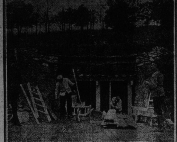
The above view shows a specially constructed shelter for storing shells behind the front lines. Two thick covering layers of earth are interposed between the magazine and the general level of the country around in order to lessen the risk of explosion should a chance shot strike the roof. The whole of this protective covering is carried on stout balks of timber and iron girders. The actual storage place is seen in the cavity behind the soldiers in the foreground.
