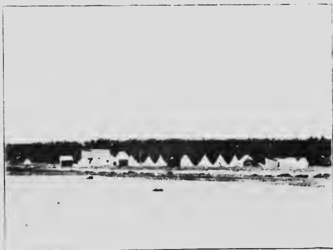
ECLIPSE CAMP, LOOKING TOWARDS NORTH-WEST.
