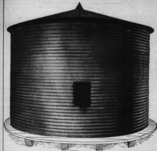
Our granary is made of heavy galvanized corrugated steel, and while stronger than the ordinary wooden granary, weighs about one third as much, making it easy to move.
