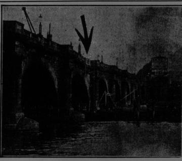
The famous Waterloo Bridge in London, England, is closed for repairs. The bridge actually started to sink as may be seen in this photograph. As a result other bridges in London are overloaded with traffic.
