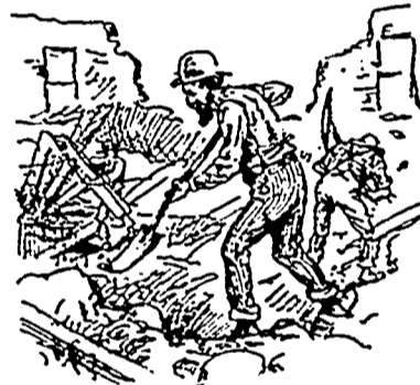
"I was helping dig out the cellar"
