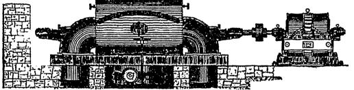
HE accompanying of shows the direct on nection of two 20" Crocks TI RBINES under 50 ft. ber to ELECTRICAL GENER ATOR at power station North Shore Power Co., St. Narcisse, Que.
