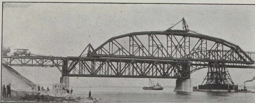
One Channel Span of the St. Lawrence River Bridge Moving Into Place.
