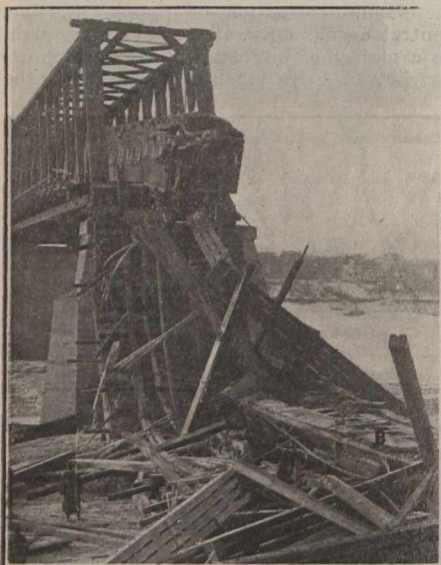
Wreckage of the Timber Truss.
