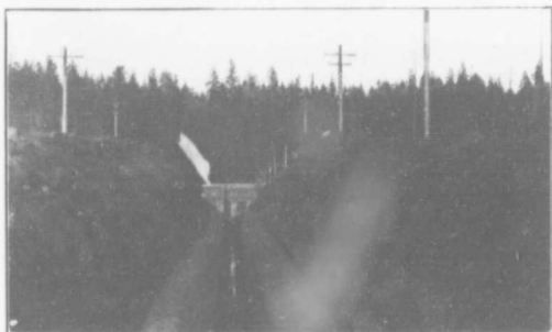
Pipe Line to Power House
