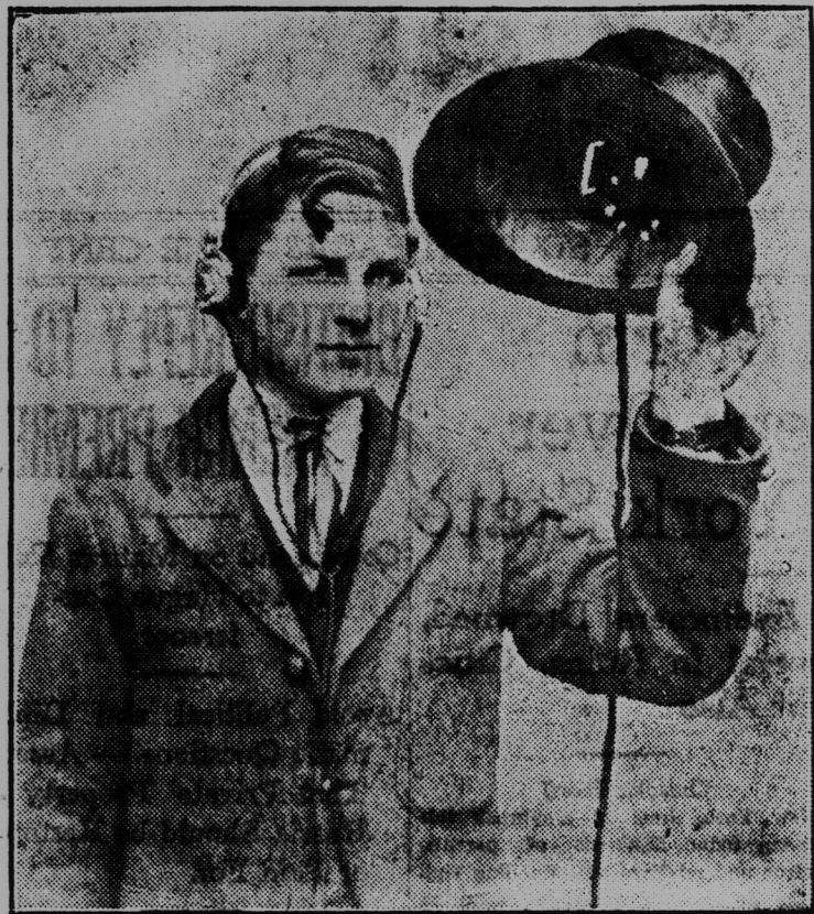
The wireless outfit is so constructed as to fit inside an ordinary high hat (sometimes called a stove-pipe), and has a wave length of 850 to 5,000 metres. The photo shows H. Day, an English youth of 18 years, who built this novel outfit.
