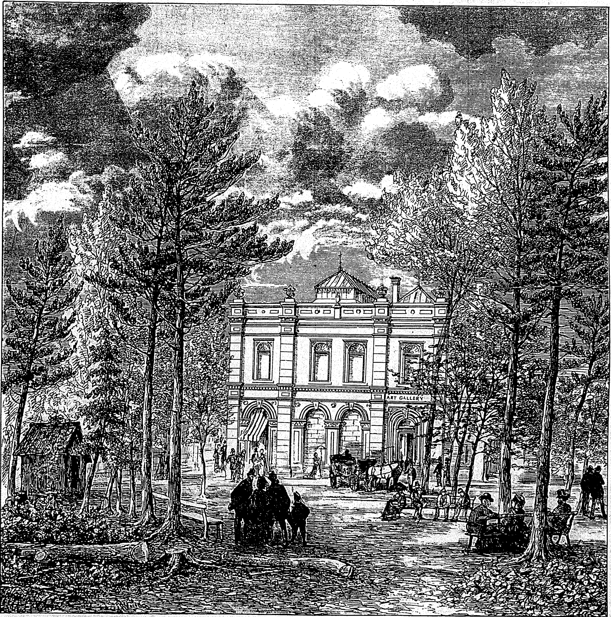
VIEW OF THE ART ASSOCIATION BUILDING, PHILLIPS' SQUARE, MONTREAL.
