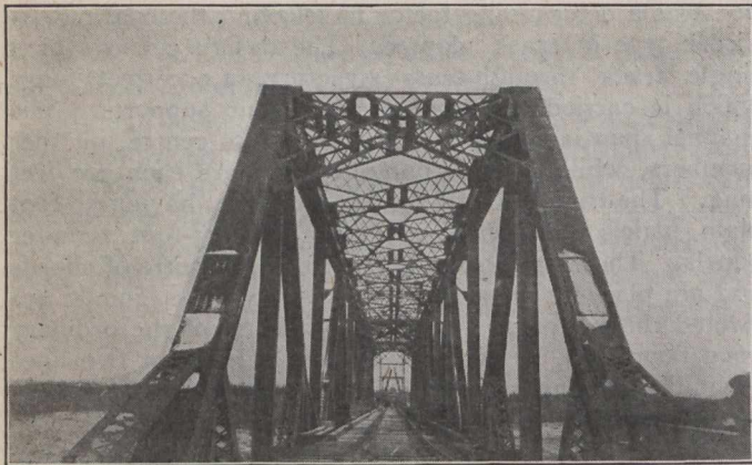
Portal, Looking North
