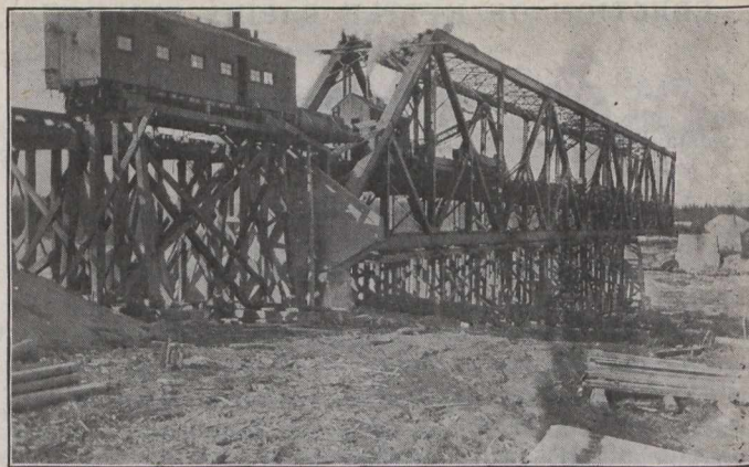
South Flanking Arm in Place; Cantilever Erection
