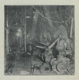
Twenty-seven Cameron pumps were used on the Mount Royal Tunnel, the one illustrated is shown working against a total head of 290 feet.
