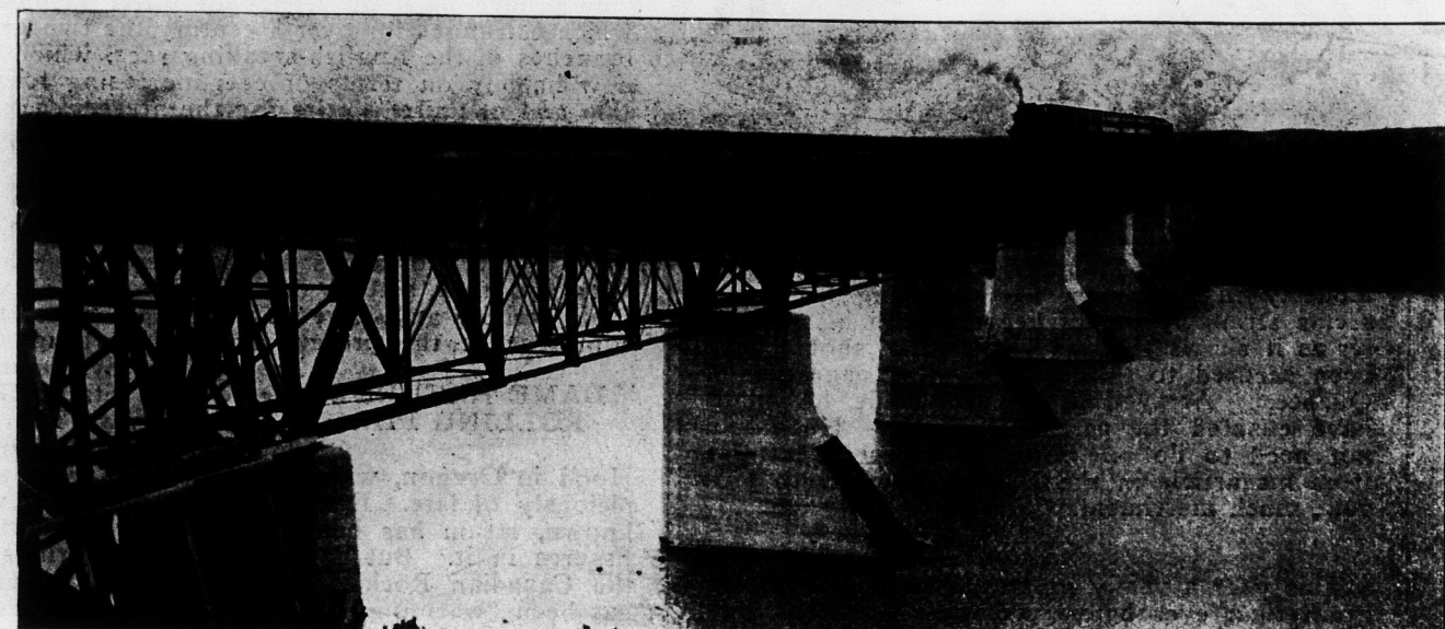
Bridge over Saskatchewan River, near Battleford, Sask., on the C. N. R.
