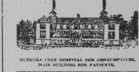
MUSKOKA FREE HOSPITAL FOR CONSUMPTIVES. MAIN BUILDING FOR PATIENTS.
