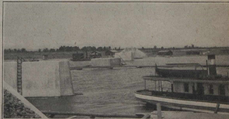
Foundations complete, looking north.
