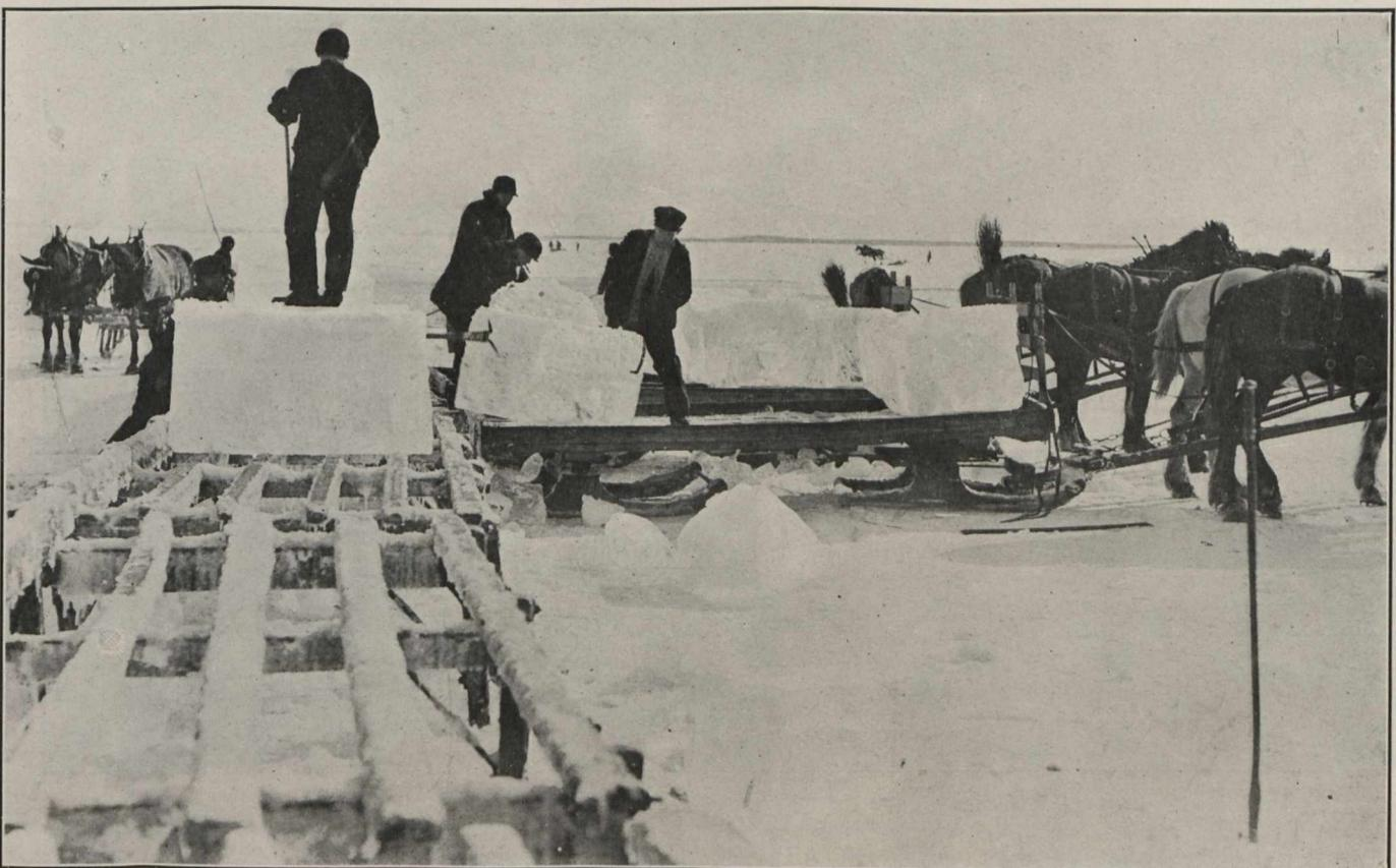
**Transporting the Blocks** Twenty thousand such blocks as these, each 48 inches long, 22 inches wide, and 28 inches thick have been used in the construction of the Ice Palace, the total weight of which is about four thousand tons.
