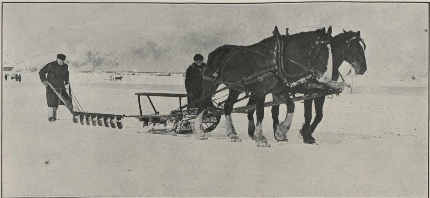
**Laying Out the Field** A sort of plough is used to mark off the huge squares, which are then sawed up into suitable sizes for handling.
