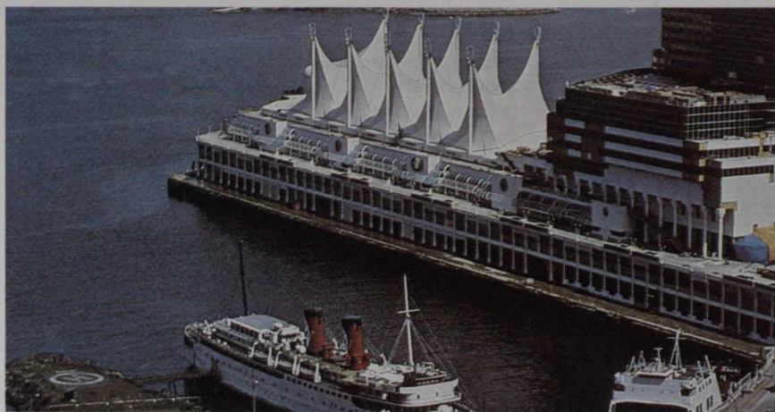
Canada Place — several buildings in one.
