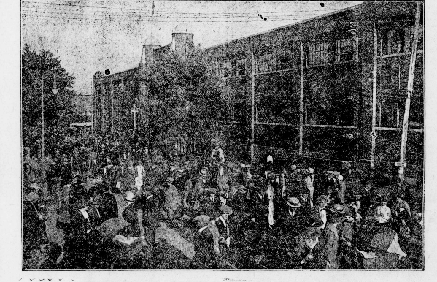
The New Manufacturers' Building, Filled With Canadian Products.
